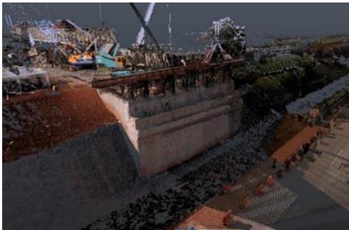
Figure 2. 3D Scanning results on Abutment
