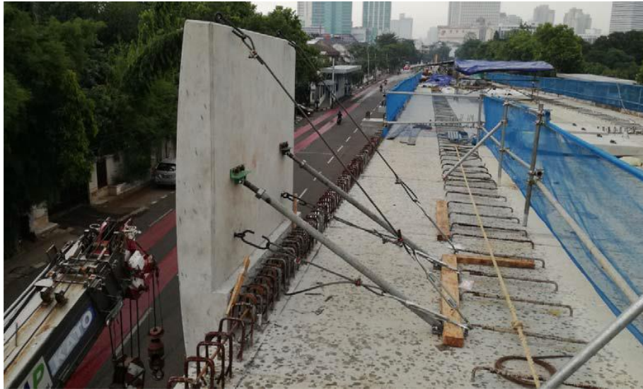
Figure 1. Precast Parapet Panel Installation (OSJ-JV, 2017)
