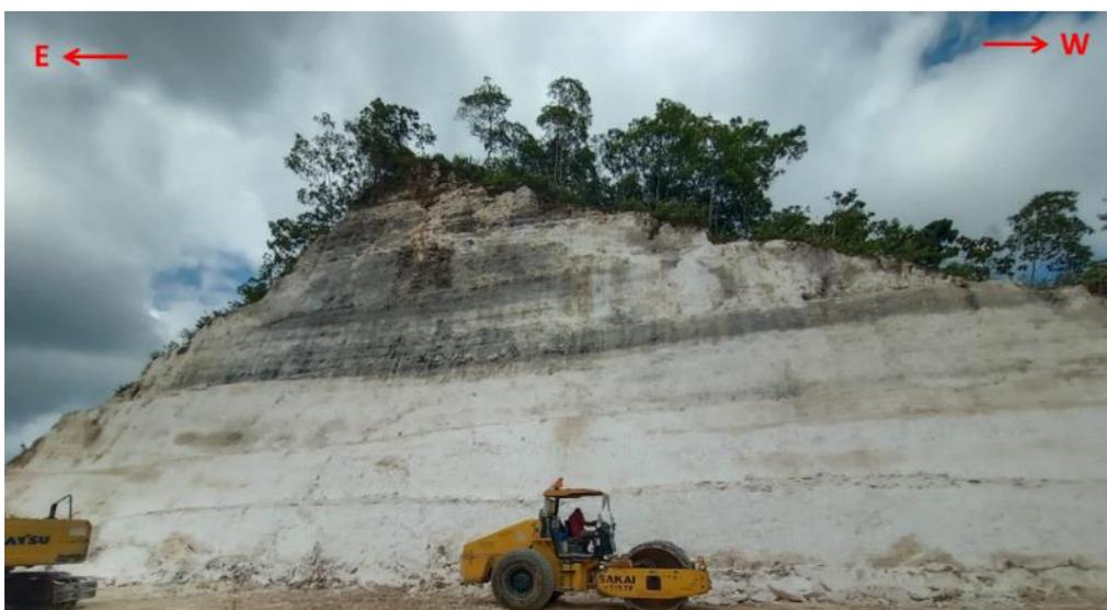
Figure 3. Condition of floatstone rock mass structure (slope facing north): moderate weathering level, type A rock mass structure and composition, good rock mass condition, GSI value 45-65
