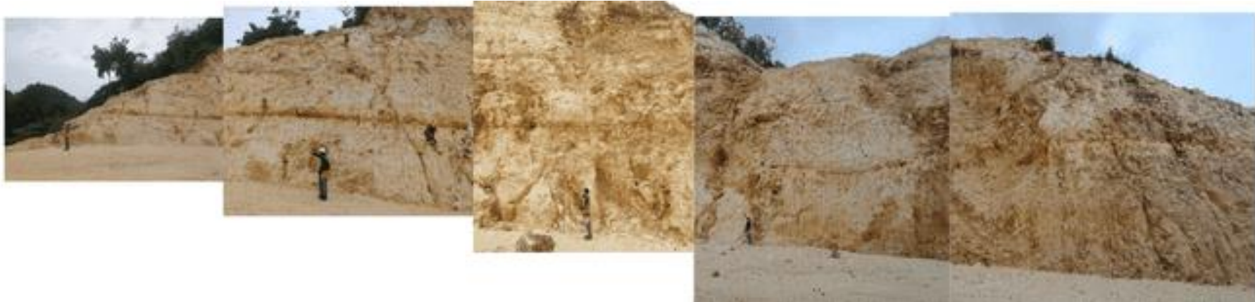
Figure 2. Slope outcrop STA 8+400 to STA 8+500
