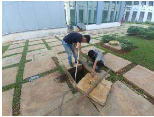
Figure 3. Cleaning Process of Sedimentation Tank
