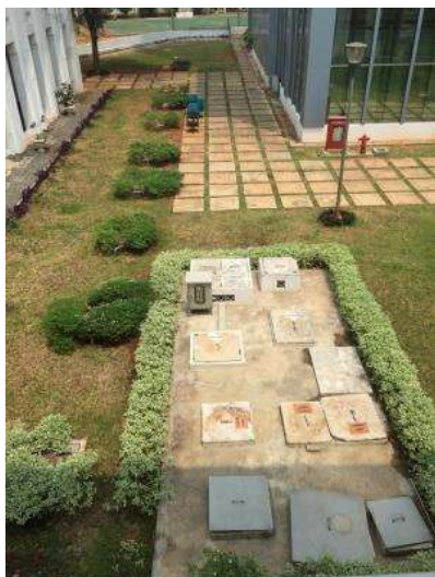
Figure 1. Location of IMERI Building's WWTP
